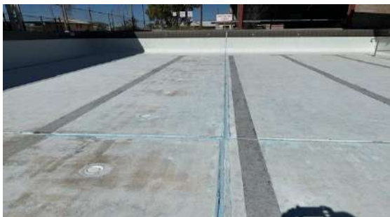
New expansion joints (Blue lines)
