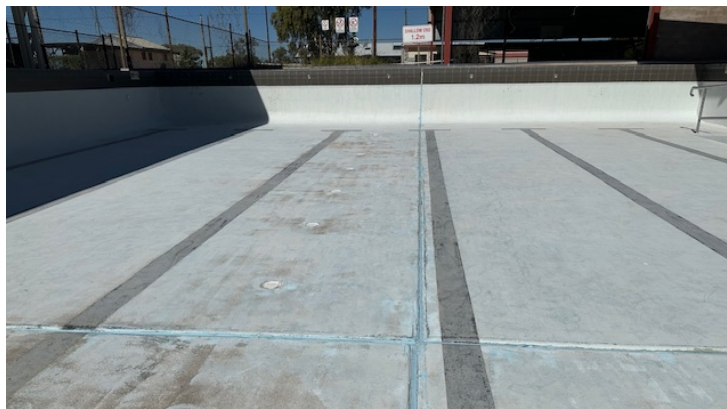
Expansion joints replaced (in blue)
