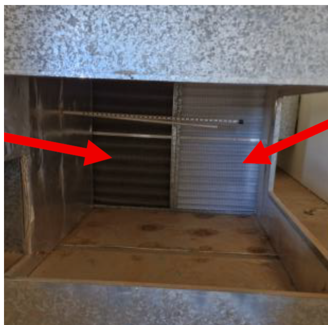
View inside air-conditioning during cleaning
