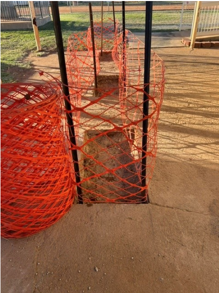
Trip hazard removed in Preparation for new concrete.
