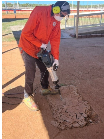
Trip Hazard removal.
